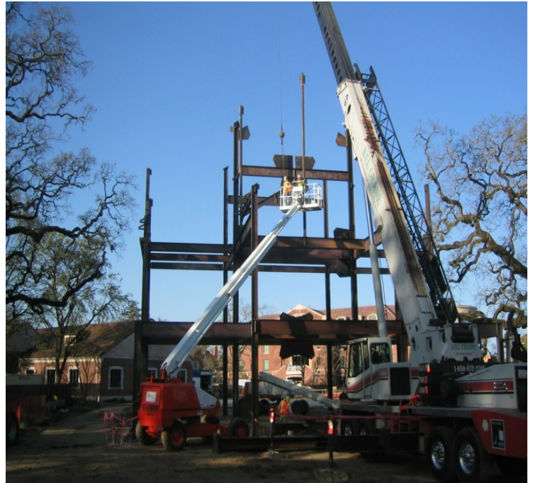
Above: Single crane and crew at work during erection
